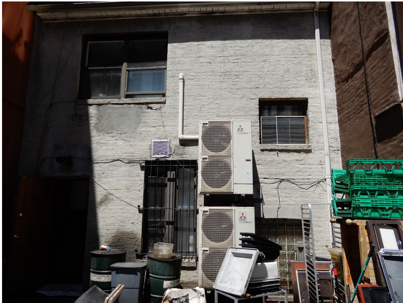
Rear Façade 2 nd & 3 rd floors
