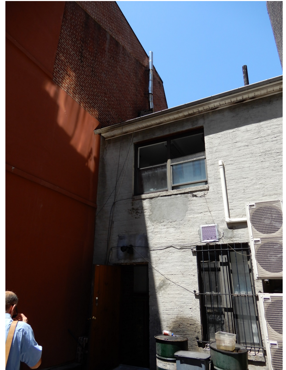
Rear Façade and Adjacent Looking South
