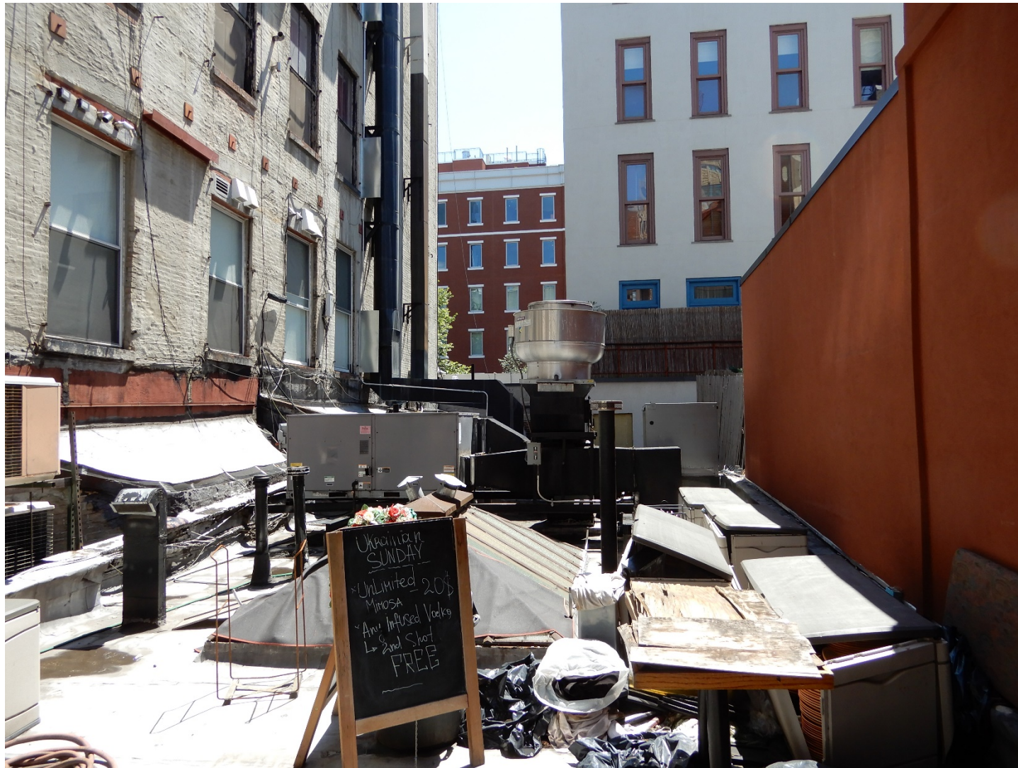
Adjacent Rear Facades Looking North
