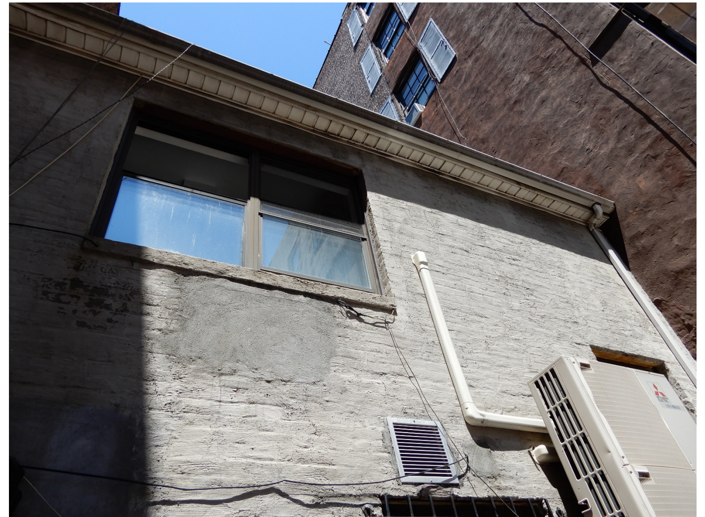
Rear Façade 3 rd floor
